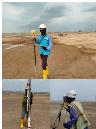
Gambar 2. Pengambilan data settlement plate dan timbunan aktual
